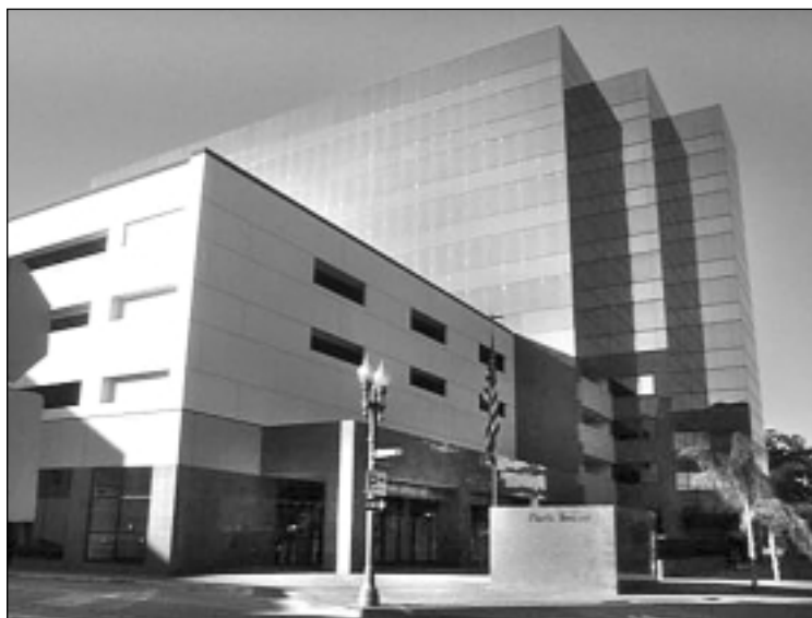
Park Tower is located at 200 W. Santa Ana Blvd. across from the Old Orange County Courthouse.
